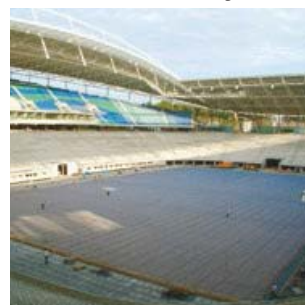
Undersoil pitch heating
