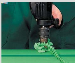
Drilling through the pipe wall
