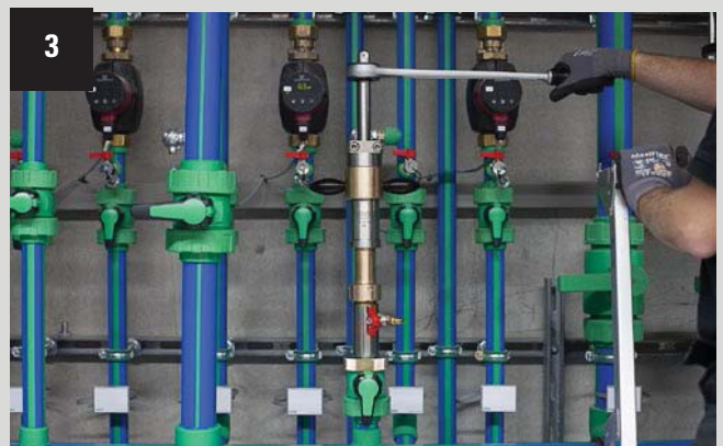
3. Start of the drilling process
