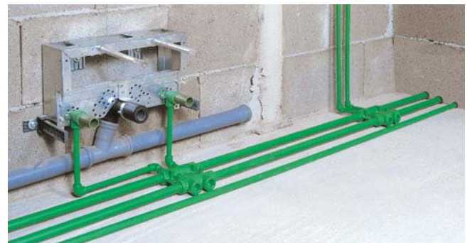
Floor distribution with distribution blocks
