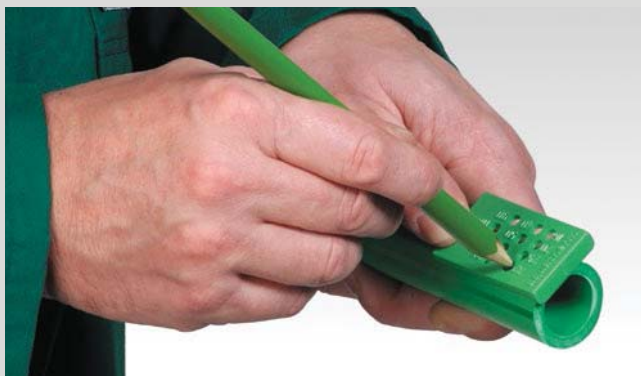
Marking of the welding depth
