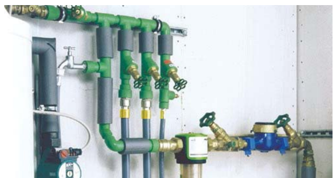
House connection station
