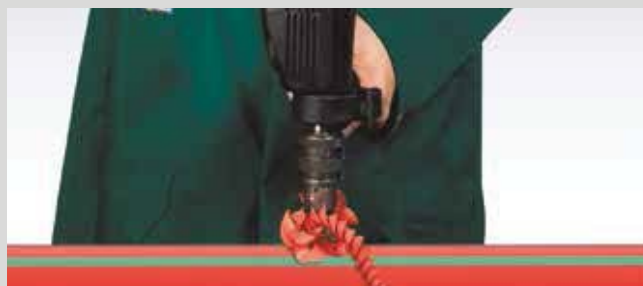
Drilling through the pipe wall
