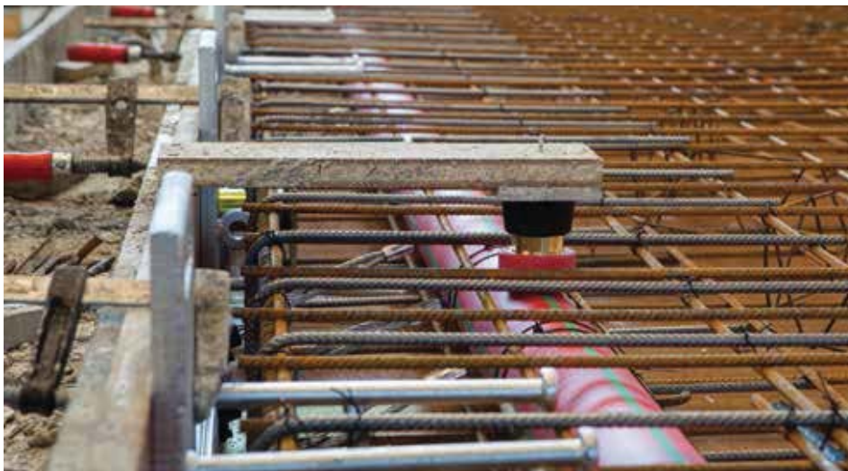
Prefabrication concrete wall
