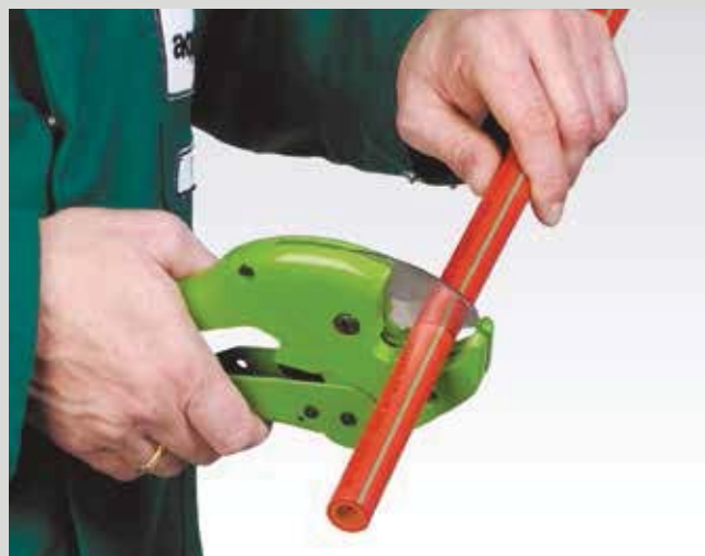
Cutting of the pipe
