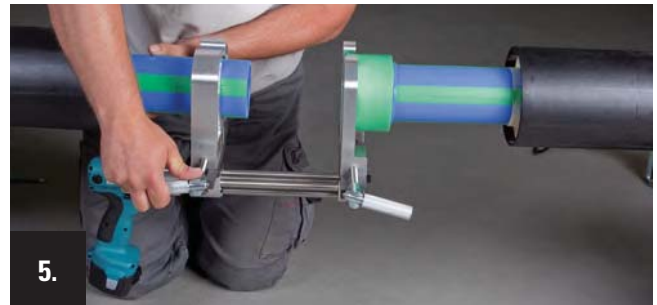
5. Pull the pipe end up to the end of the clamping mark into the welding jig and tighten the clamping jaws with the fixing screw.
